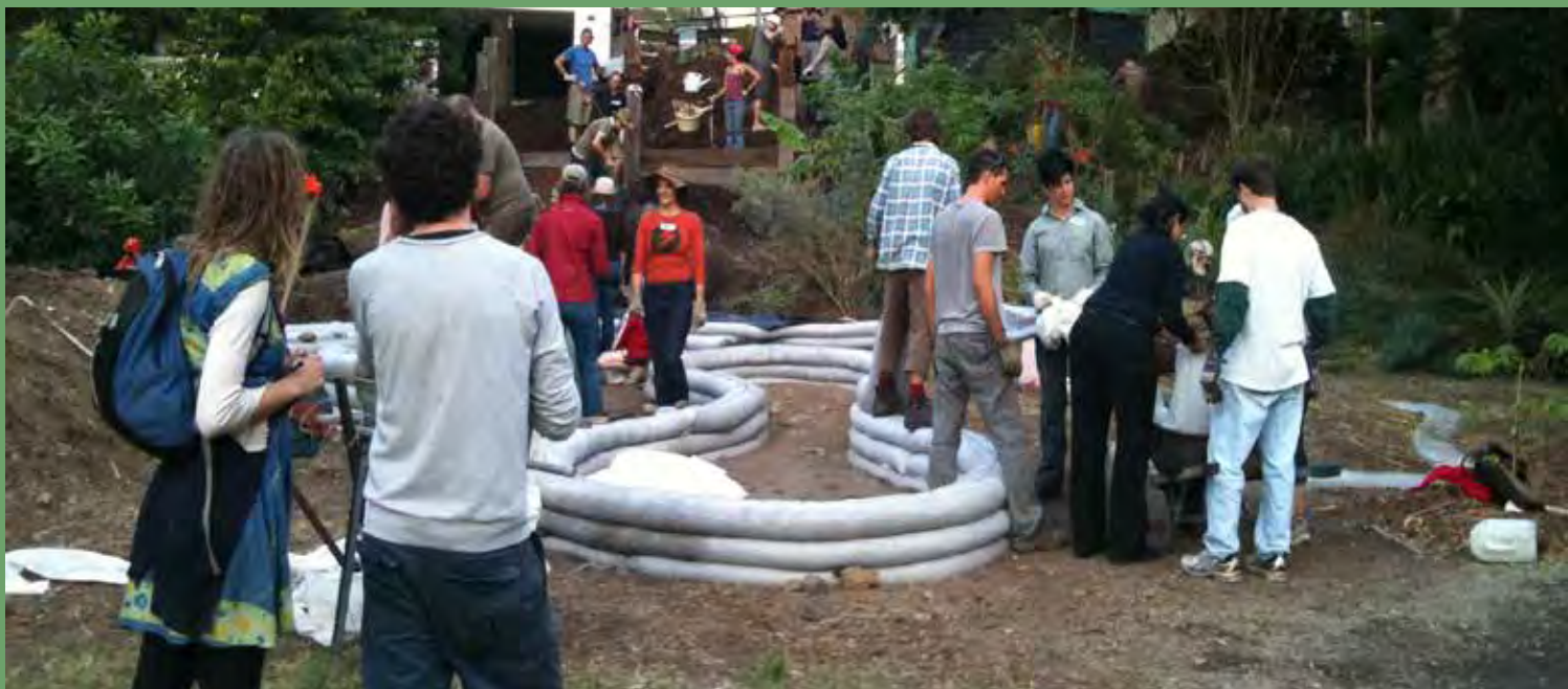
Residents building raised planters using low technology solutions
