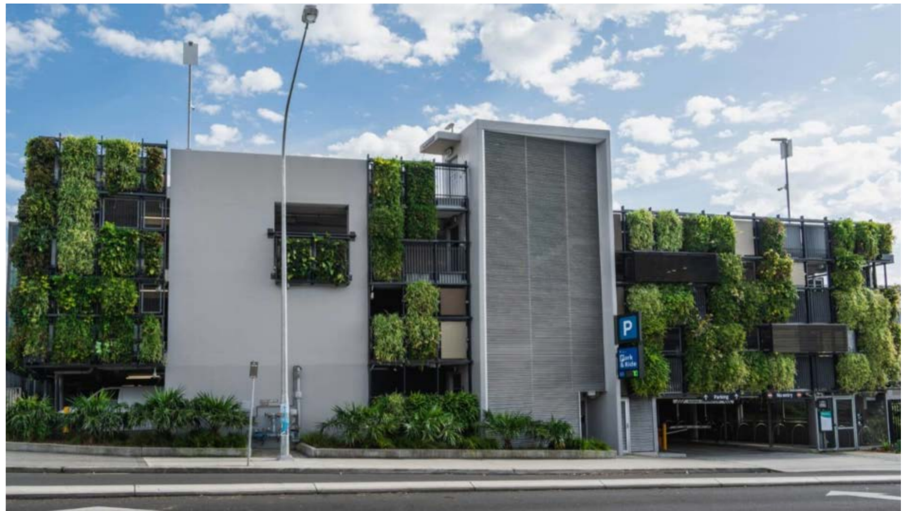
Example of a 'green' multi-storey carpark
